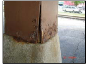
TREAT BASES OF COLUMNS AND REPLACE METAL PLATES
