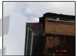
WOOD ROT REPAIR AND RESTORATION
