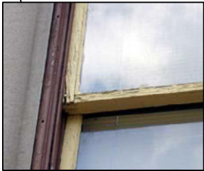
WINDOW REPAIR AND RESTORATION
