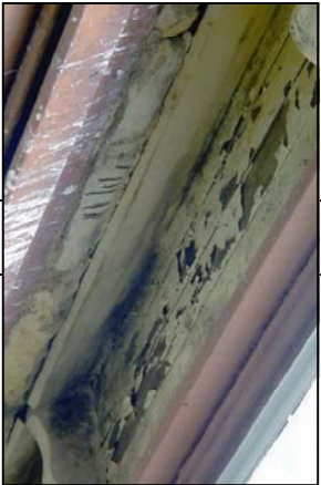
WOOD ROT REPAIR
